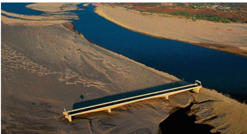
Choluteca Bridge after Hurricane Mitch on Choluteca river
